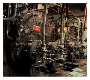
Industrial pipes and boilers run boiling water continuously 24-7 so within a few weeks or months the pipes and boilers become so clogged with serious mineral deposits (scale) on the sides of the pipes and boilers that it interferes with the efficiency of the systems.
